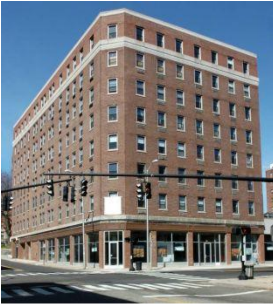
Apartment building at 144 Golden Hill St
